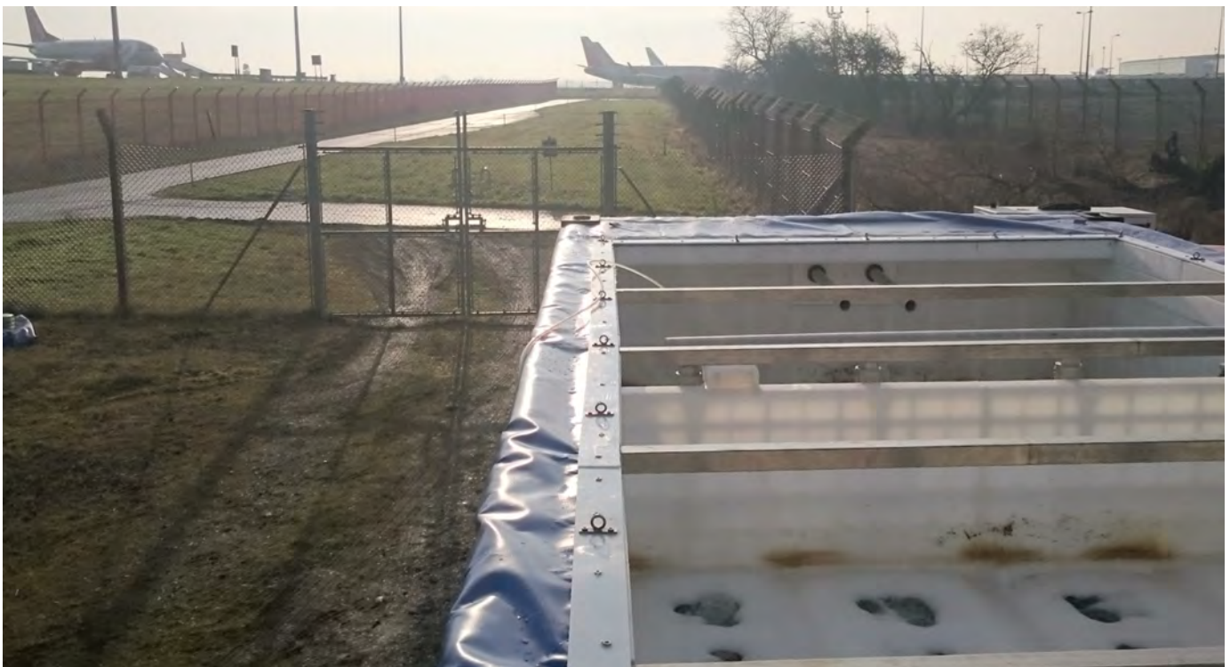
BioContainer 20' BioMax in operation
