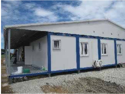
Construction Site Office
